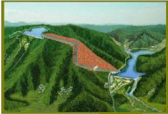
PUMPED STORAGE POWER PLANT (50MW)
