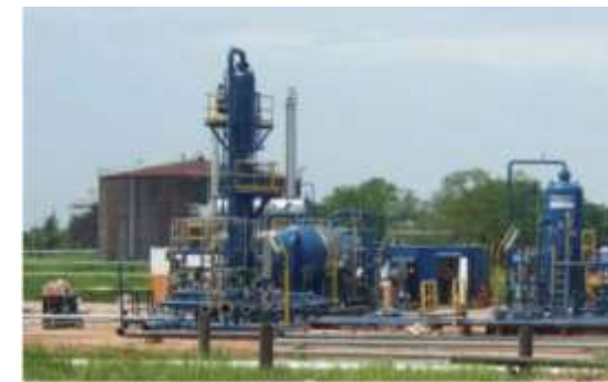
Modular Construction Techniques deploying skid mounted units
