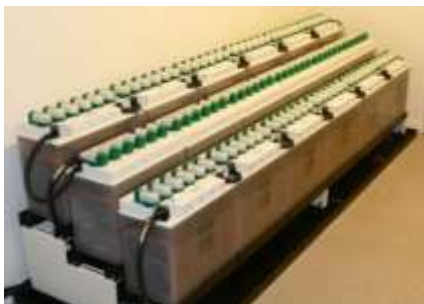
Lead acid batteries
