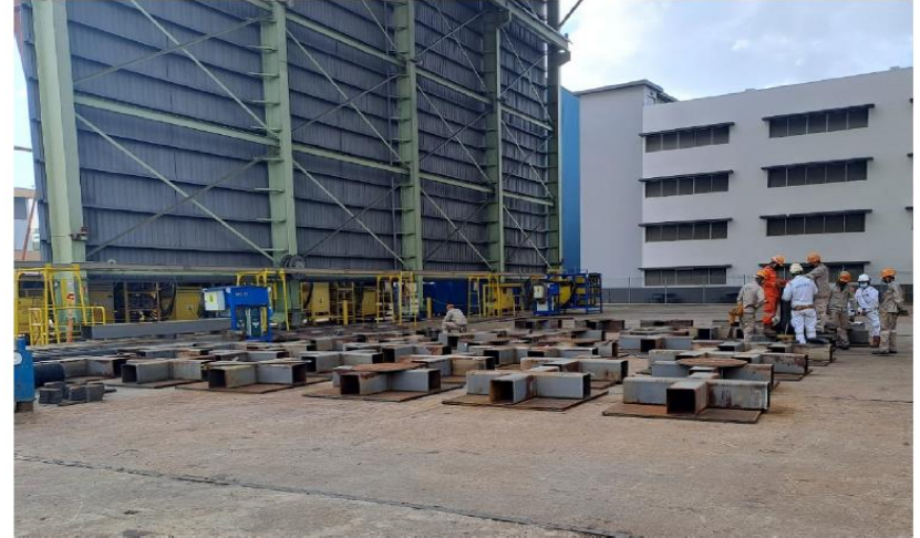
Temporary Supports Fabrication
