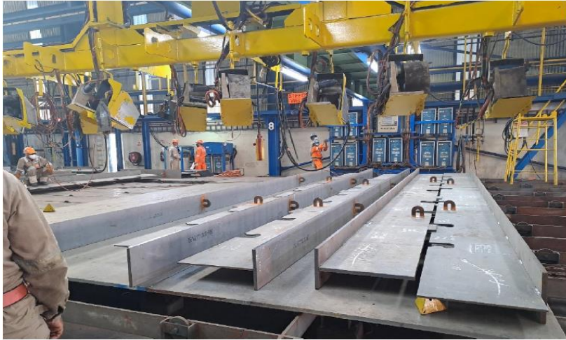
Fabrication of T-Bars for under deck
