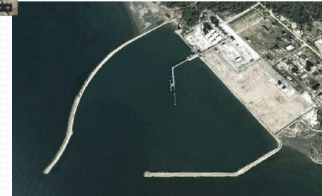
THE "VLORA-1" PETROLEUM PORT
