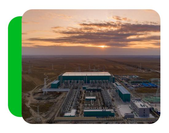
World's first four-terminal ring power network based on VSC-HVDC technology. The project includes the construction of four  $\pm 500 \text{kV}$  converter stations, with a total converting capacity of 9 million kVA and a length of 666 kilometers.
