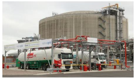
A conventional LNG import terminal needs a "trucks loading facility" to allow ssLNG export for different applications
