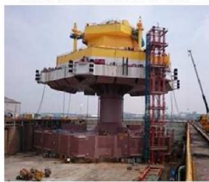
The floater lost control and leaned on 9 May
