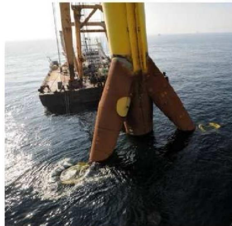
Tripod foundation lowered to seabed
