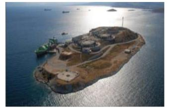
Today, the Terminal has the capacity to accept and handle some 5.2 -5.3 billion m3 annually. More specifically, following an expansion of the infrastructure and upgrading of the facilities SMSR gasification capacity to 1,000 m3/h of LNG from 271 m3/h LNG previously and the peak gasification has increased its capacity to 1,250 m3/h from 500 m3/h LNG.
