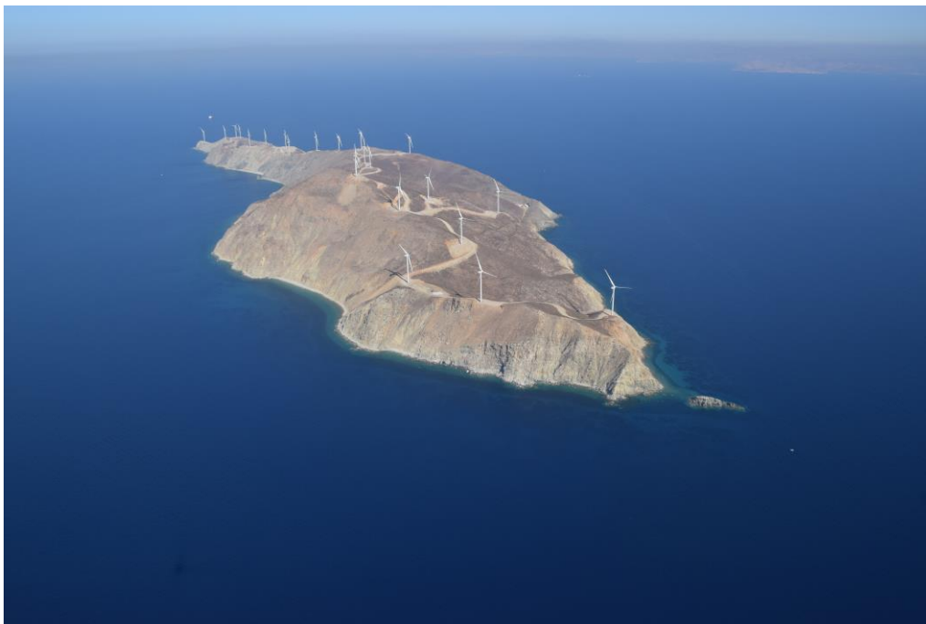
One of TERNA's latest wind projects on the rocky and uninhabited islet of St. Giorgio, located south west of Cape Sounion in the Saronic Gulf with 70 MW of installed wind capacity. Electricity produced at St. Giorgio is channeled via a 20 km underwater cable to the mainland grid.
