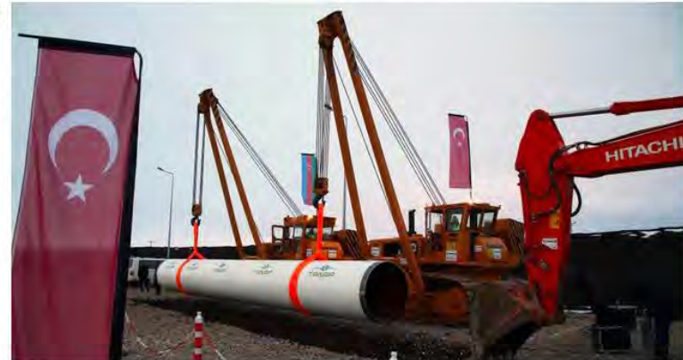
The Trans-Anatolian Natural Gas Pipeline (TANAP) will bring natural gas produced from Azerbaijan's Shah Deniz-2 gas field, and other areas of the Caspian Sea, primarily to Turkey, but also on to Europe.
